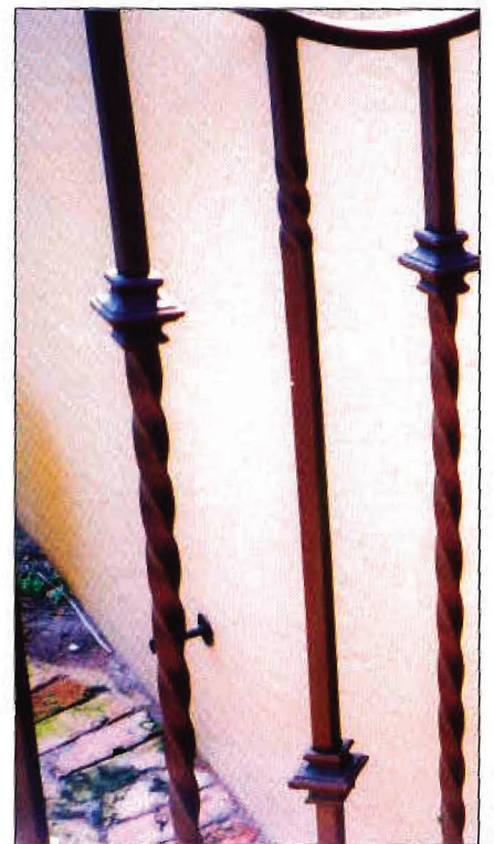
This aluminum rail with marine grade aluminum cast collars also shows a coherent coating in excellent condition after three years on Florida's Intracoastal Waterway.
