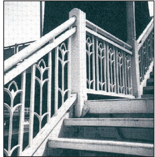
FIGURE 4: The original panels, which adorn a bridge in Pennsylvania.
