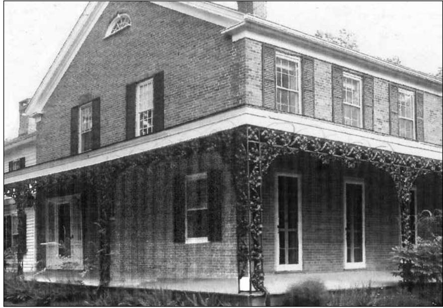
Four different cast iron designs had been fabricated as a veranda onto a house originally built in 1806. The project meant making aluminum replacement pieces based on the cast iron originals.
